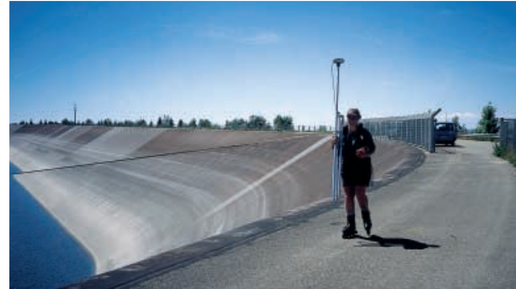
The Hornberg reservoir: surveying this vast structure in the southern Black Forest using the GPS stop&go technique.
